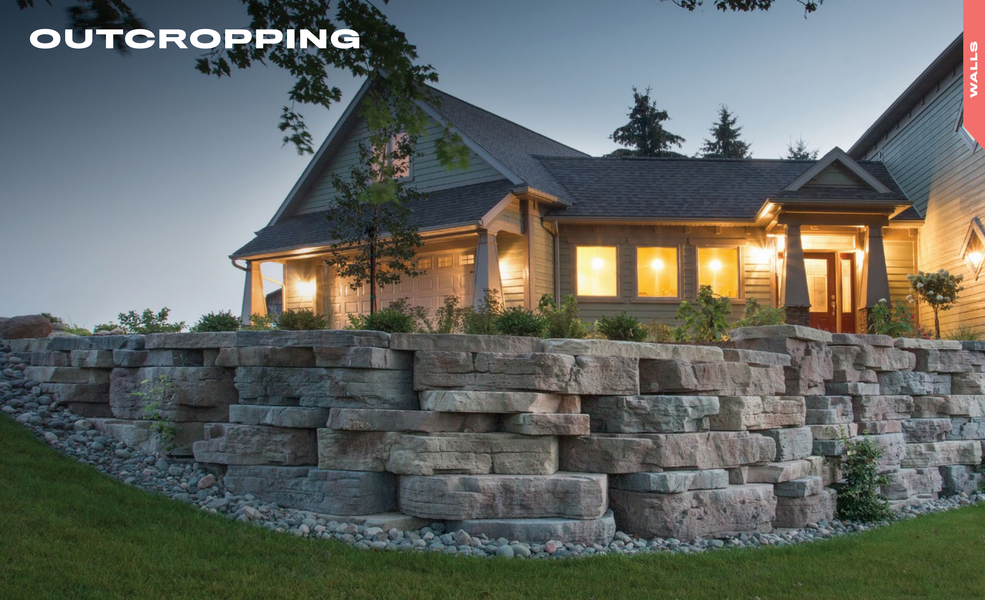
Outcropping Wall in Lakeshore Blend using Irregular Steps as Coping
